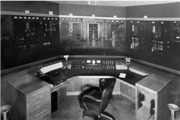
**The WE 407-A4 as installed at WTOP (then JSV)**
