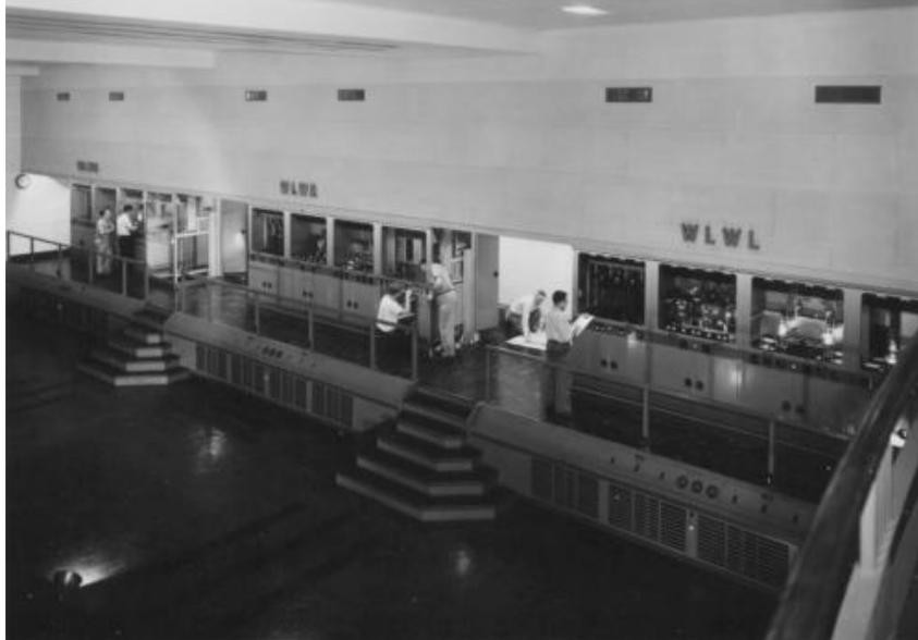
The three transmitters on the east side of the concourse were complete transmitters while the three on the west side were RF sections only – utilizing the power section and modulator of the transmitter on the opposite side.
