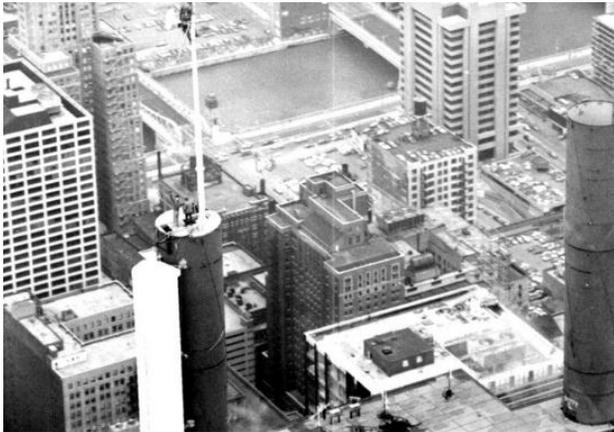
The antenna for WLAK 93.9 being mounted at the top of the 40-foot pole. Note the top of the East cylinder was open, with TV 7 and 11 side-mounted on the base.
