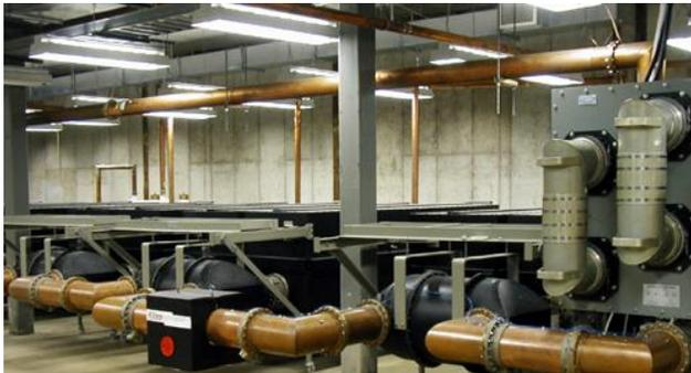
This line begins with 3-inch rigid line and ends up 9 stations later with 9-inch EIA rigid line connected to a large 9-inch EIA patch-panel. That allows the combined power of all stations to be directed to either upper or lower 6-bay antenna if either half of the transmission line or antenna system fails.
