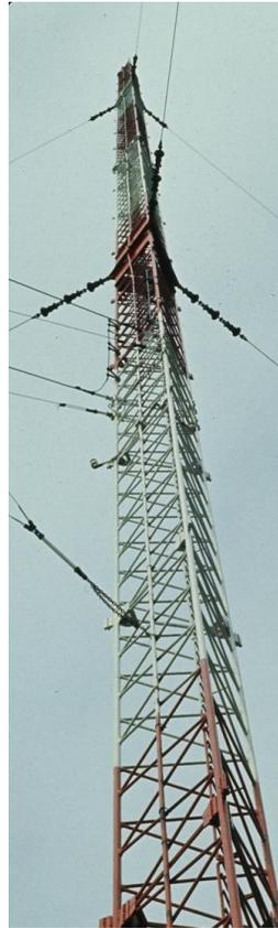
KSL used its new corporate structure to continue to improve facilities in Salt Lake City, upgrading their transmitter system from a shunt-fed antenna to a series-fed 192 degree tower in 1976, and a new transmitter building in 1985. A new Nautel Ampfet 50 was installed, serving until the installation of a Nautel XL-60 in 2005. And now, in 2012, KSL reports the installation of a Nautel NX50HD to carry it into the future.
