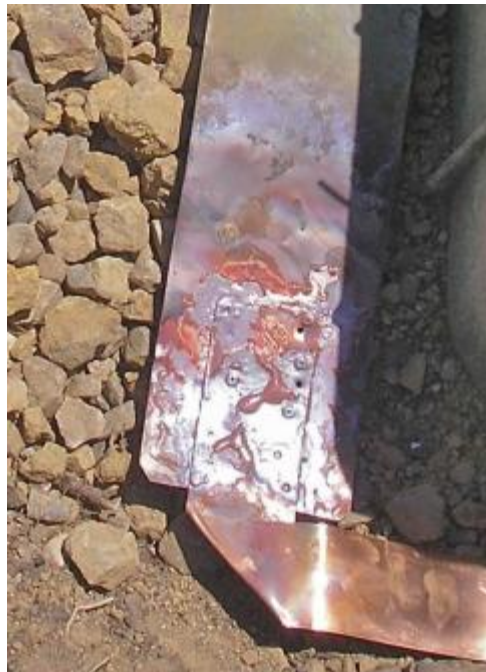
Brazed joint after copper pop rivets were installed. Yes, we ran out of 4-inch strap.
