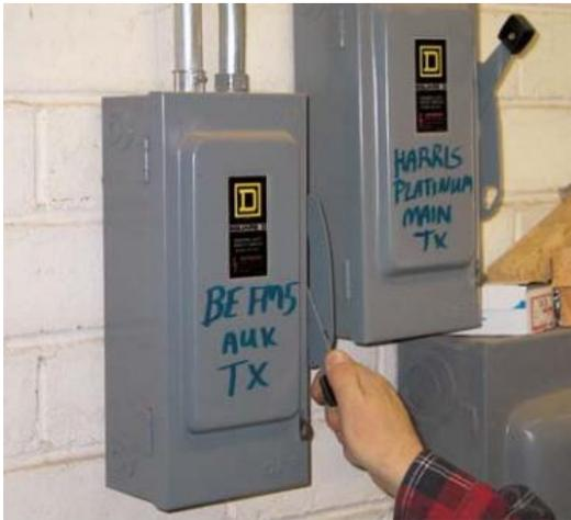
There are some transmitters that do require multiple power sources. I know; I maintain one: a Harris FM-10K. There is a 3-phase power source, and a single-phase power source. In other words, two different circuit breakers.
