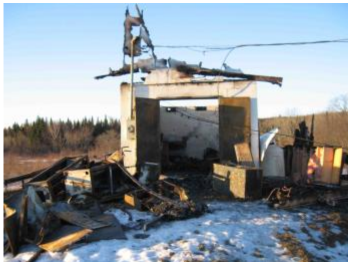
This is an ex-Transmitter Building.
