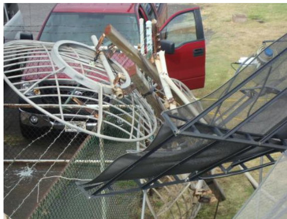
A nasty storm caused two STL dishes to fall down through the satellite receive dish
