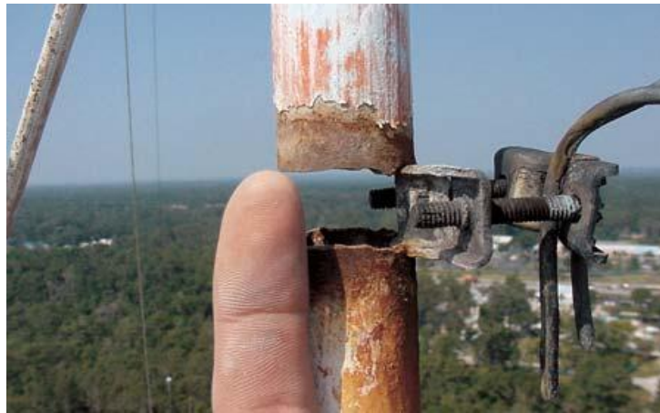
This tower leg was not designed to have a window
