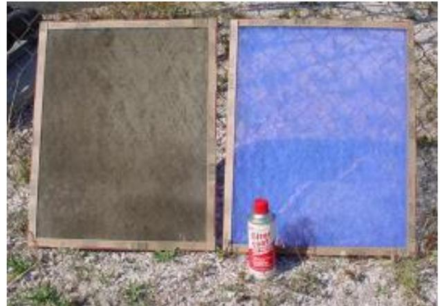
The filter on the left is shown after three weeks in typical service way up here on the dry, dusty "Plains." The filter on the right is a new filter.
