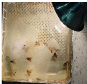
Eventually, each of the critters will hit the water and the detergent will wet their wings. None of those critters will make it over to clog the air filter on the transmitter.
