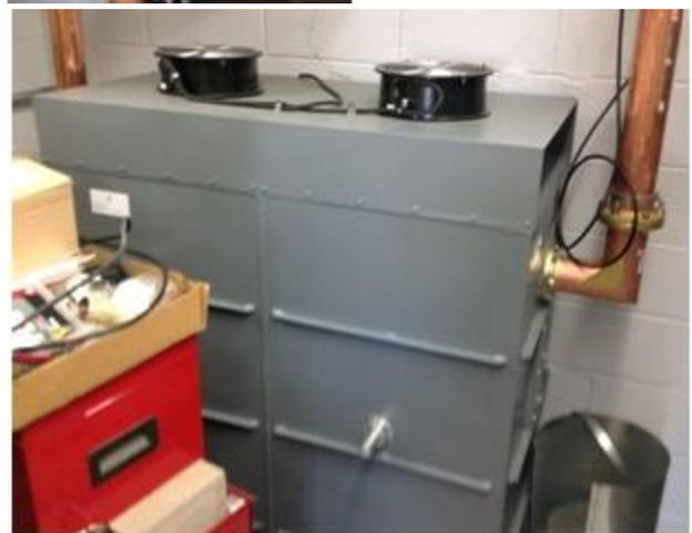
**Our new AAT 40 kW bandpass filter, plumbed in place, and ready for operation on 91.1**
