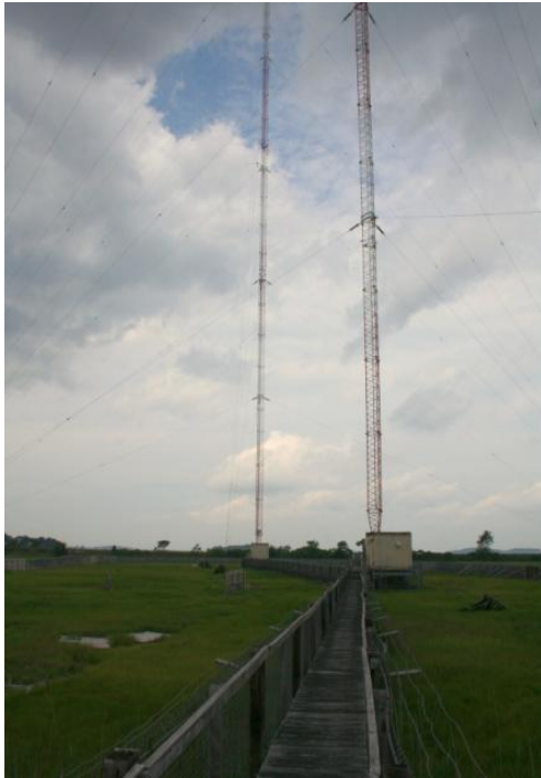
The elevated tower bases and walkways keep the tidal waters well below the towers
