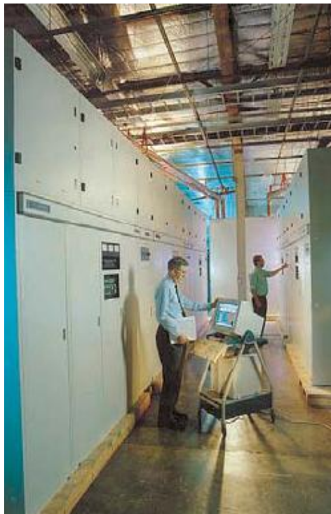
Hilmer Swanson, checking the operation of a DX-1000 (TPO: one million Watts)
