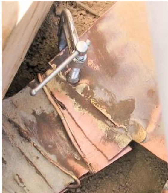
A copper “patch” is in place prior to brazing
