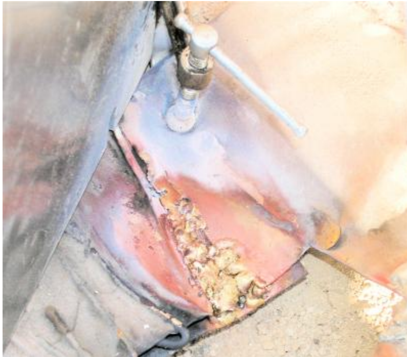
The completed repair. Caution! It is still very hot!
