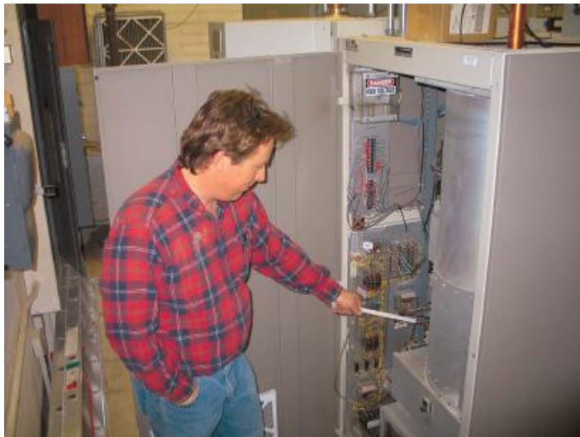
Before touching anything, ensure any power is dissipated
