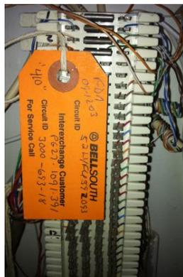
Furthermore, if your facilities have dedicated computer service lines, you should locate the service provider’s modem units and trace the lines to your demark block for identification.
